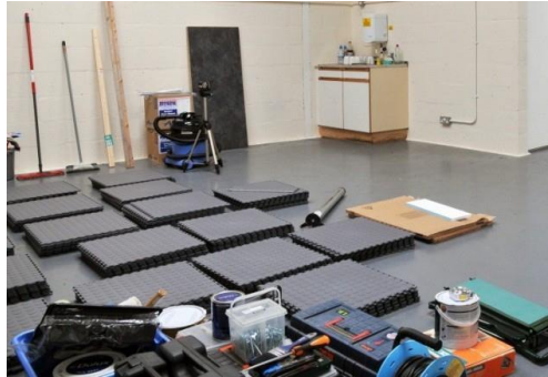
Pic 1. Break down the pallets and allow tiles to acclimatise
