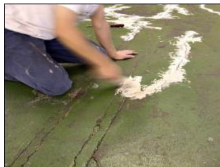
Pic 2. Sweep the floor, remove any highpoints and patch repair or level any cracks or low points.
