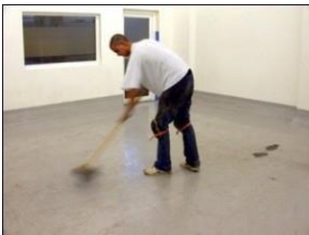
Pic 2. Sweep the floor, remove any highpoints and patch repair or level any cracks or low points.
