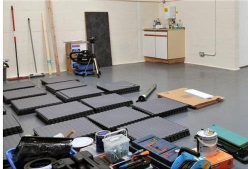
**Stage 2 – Preparation.** Sweep or vacuum the floor to remove any loose impediments. Remove any high points in the floor. Fill any holes with a rapid setting floor repair compound such as Ardurapid A46 or similar. For uneven surfaces that require smoothing use a smoothing compound such as Ardex Feather Finish.
