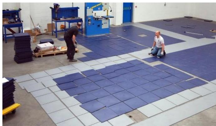
**Pic 5.** Don't force the tiles, offer up the corner of the tile and gently hammer the joints together.
